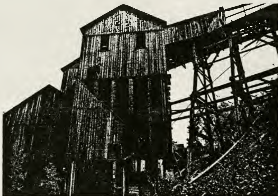
Figure 83. Revenue Mill (structure #34), north view showing new ore bins and tramway entering east side of mill.
